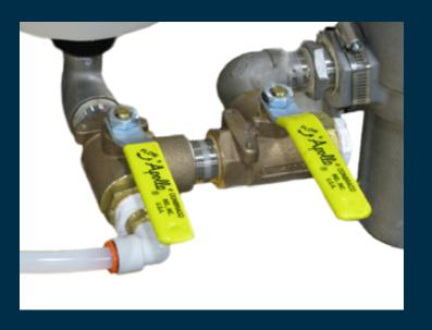
**Step 2:** Check filters periodically for clogging issues. Use a 9/16" wrench to remove the filter cap from the filter body. Remove the filter basket and clean thoroughly.
